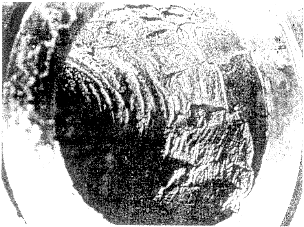
Pipe condition before lead-bismuth technology improvement program
