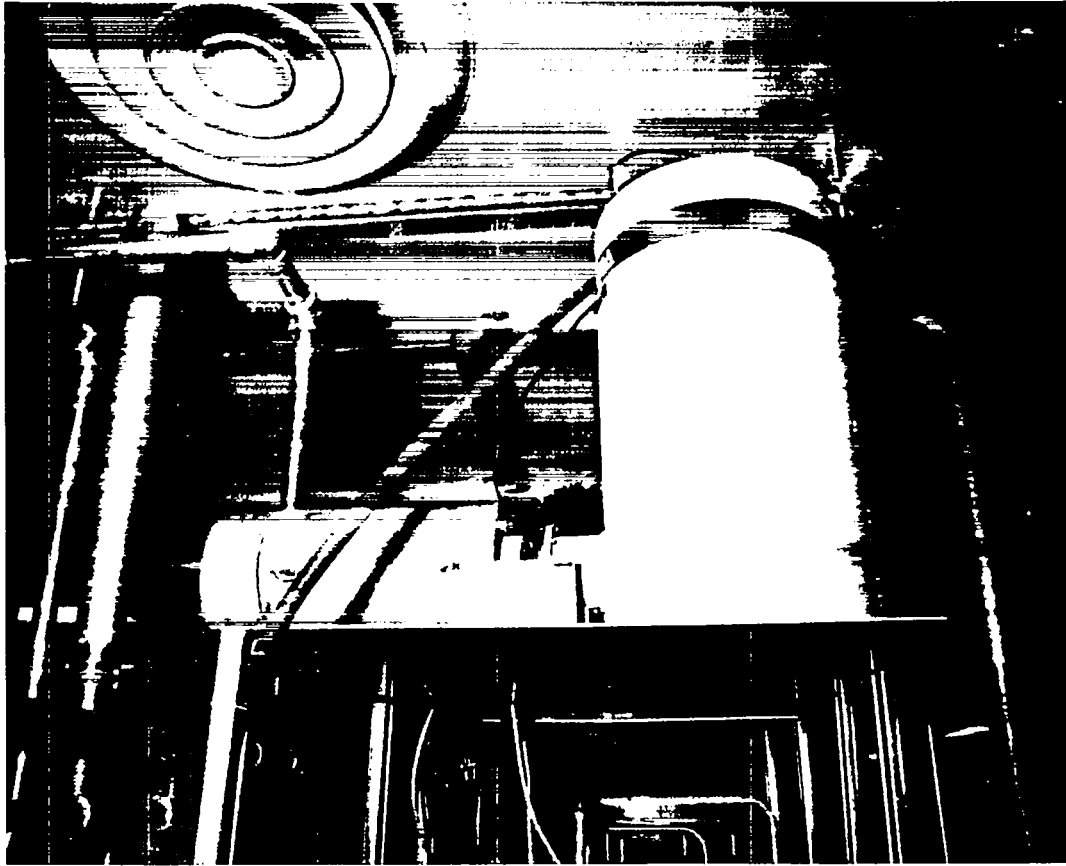
Fig. 1. High-purity germanium detector monitoring the outlet pipe from an anion exchange system at Los Alamos.
