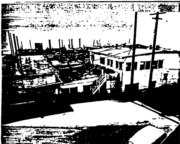
Fig. 1. The original wooden D Building which housed the chemists and metallurgists in CMR Division. Note that the chemical hoods of the laboratories on the first floor were vented individually, usually without filtration.
