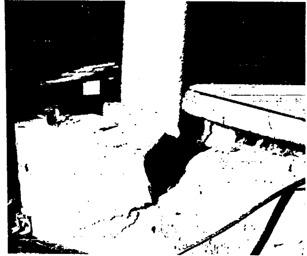
Fig. 12. Cracking at the foundation of the second structural model, Test 56.
