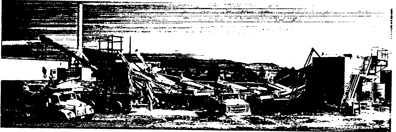
Fig. 27. Loading steel beams onto truck for disposal.
