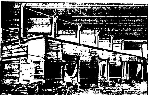
Fig. 24. Precipitron and filter area after blower room and intake plenum were removed.
