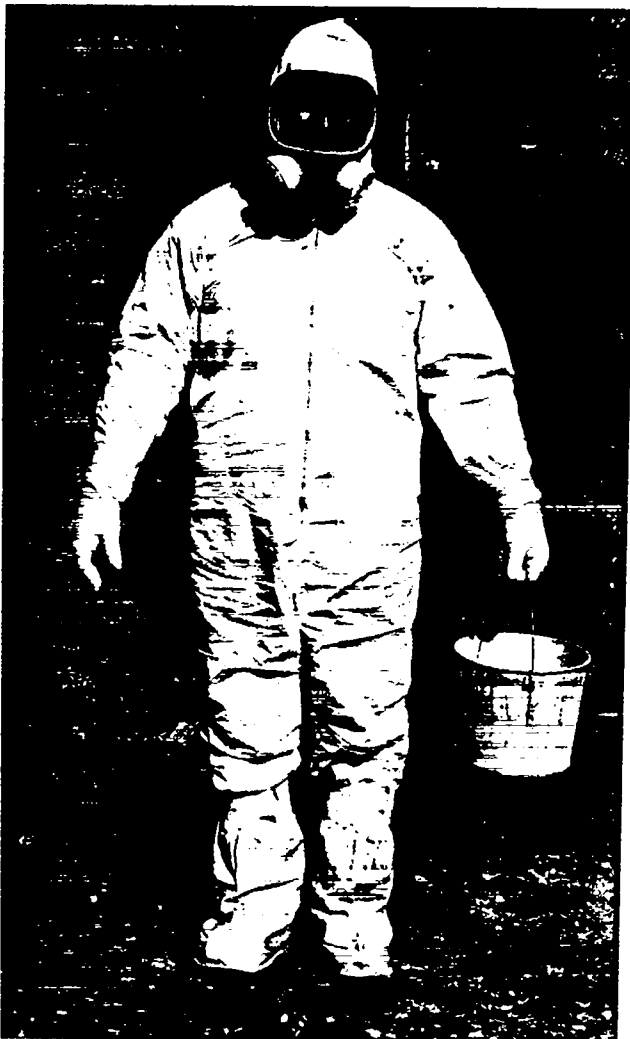
Fig. 34. Worker suited for demolition work.
