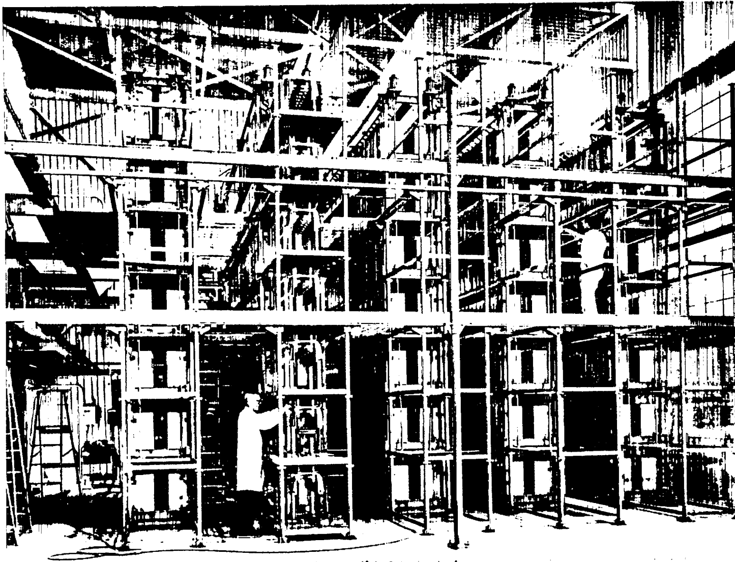
Fig. 14. Zeus capacitor bank during construction.
