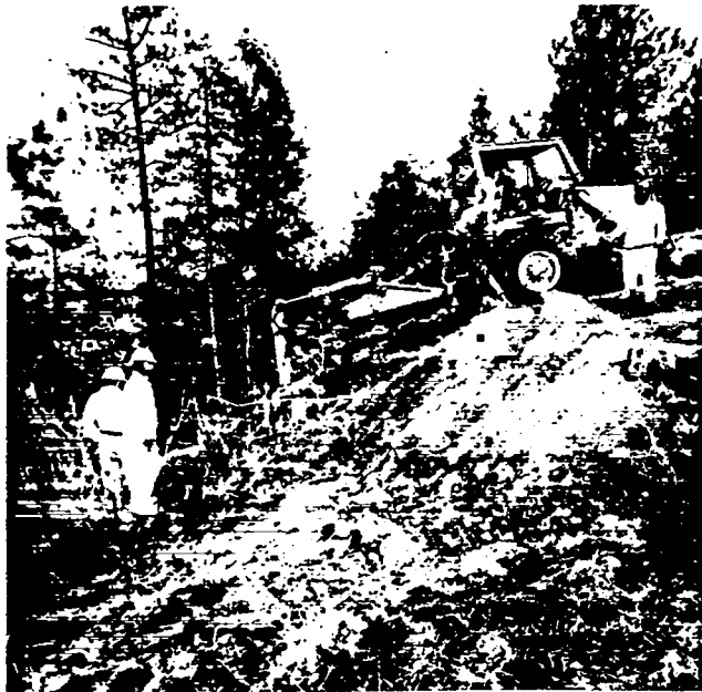
Fig. 19. Soil excavation at edge of canyon wall.
