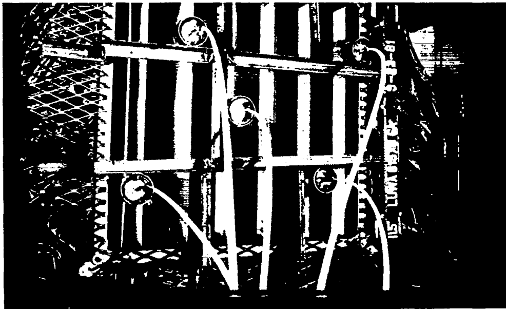
Fig. 7. Five nucleopore filter holders located just downstream of a V-type HEPA filter ready for shock testing.
