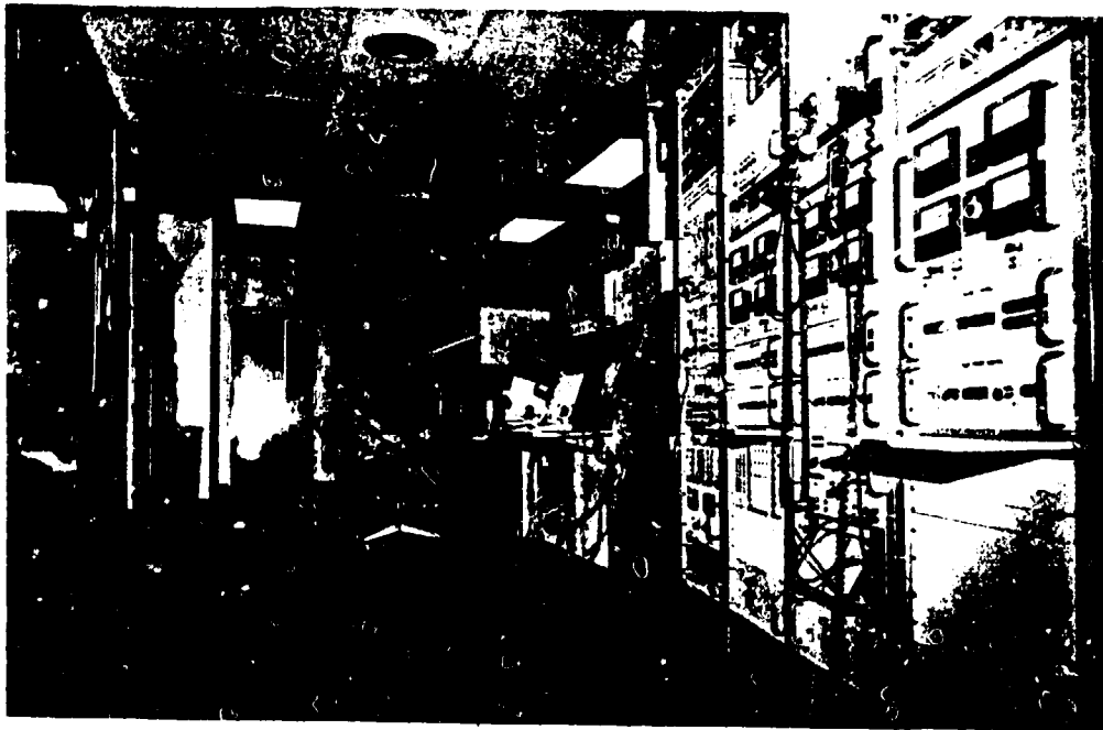
Figure 4. Helios main control room
