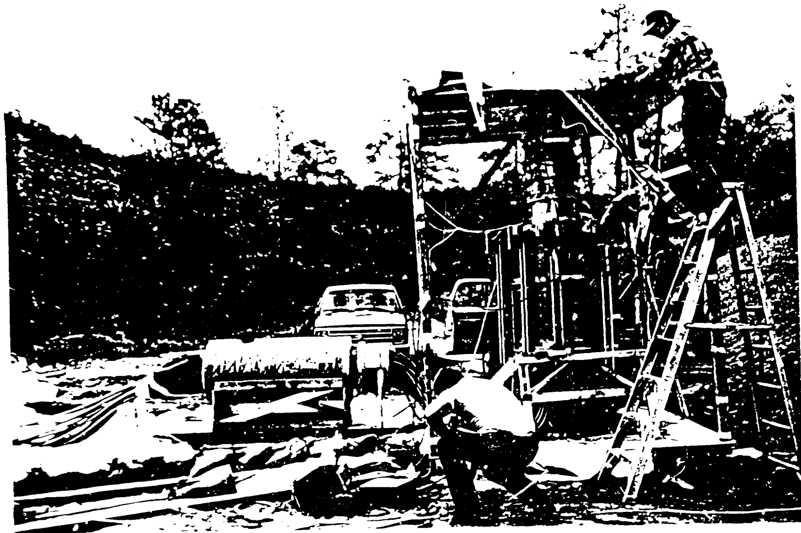
Fig. 1. The Laguna system being constructed at Firing Point 88, Los Alamos National Laboratory.
