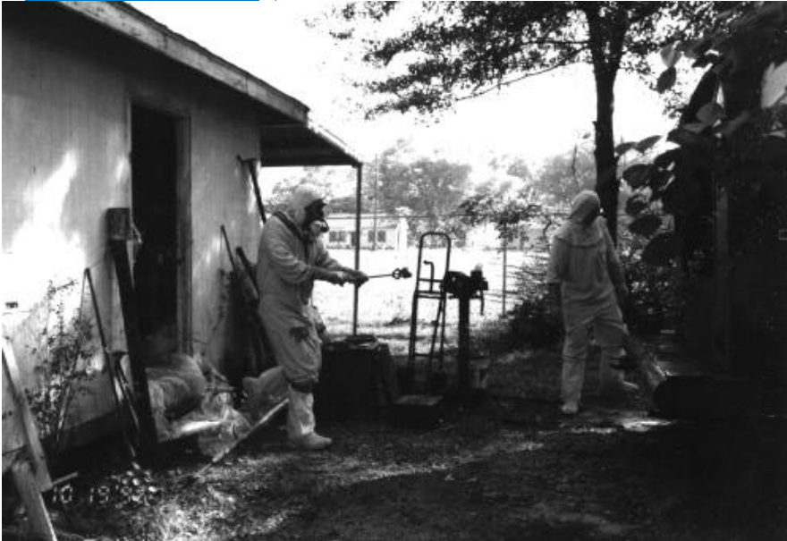
Figure 4: A leaking radioactive source used for well logging was removed after it contaminated this shed, a truck, and the well site. Los Alamos National Laboratory personnel responded to the emergency. Los Alamos is the DOE's "Lead Laboratory" for recovering the nuclear materials from such sources.
