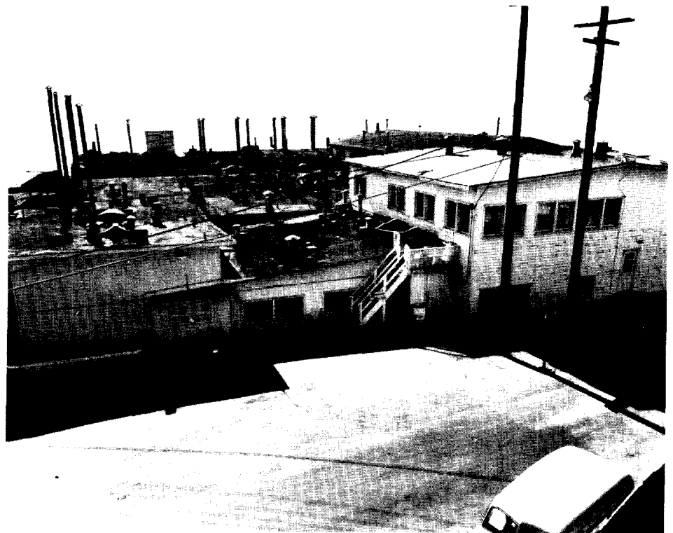
D Building, the air-conditioned wartime plutonium laboratory, bristling with separate external vents.
