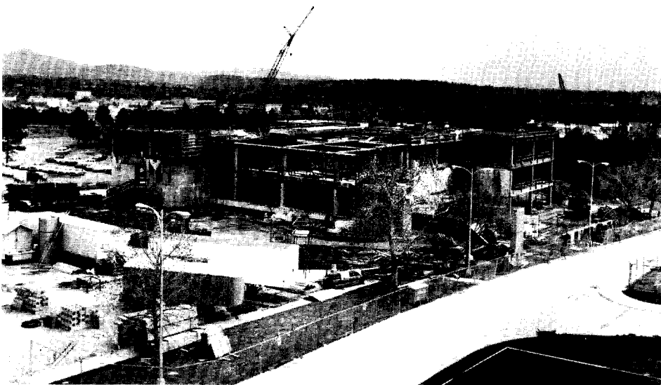
The Helios facility was constructed during the mid '70s to further explore the use of the C0 2 laser as a driver for inertial confinement fusion. Helios is an eight-beam system with an output of 10 kilojoules in 1 nanosecond.
