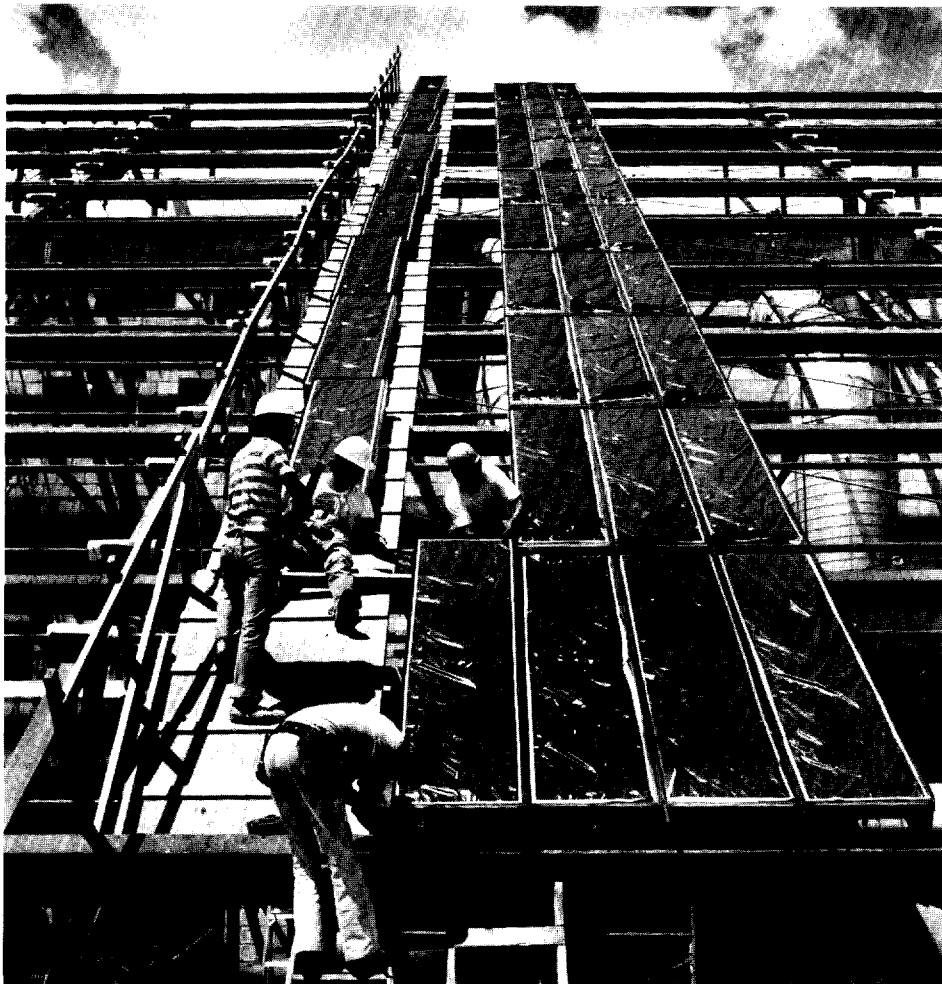
Harold spearheaded the drive for the Laboratory's National Security and Resources Study Center, shown here under construction in 1976.
