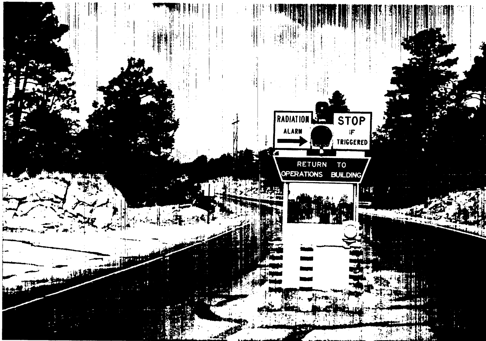
Figure 1. The guard station with alarm light and Klaxon. The system electronics are mounted inside the station.
