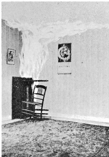
Fig. 19.11. — Pocket Incendiary operated in the space between a wall and the top of a turned-over table
