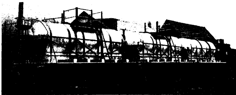
FIG. 127.—Aluminium Tank Wagons for transporting Nitric Acid. Norwegian Hydro-electric Company.
