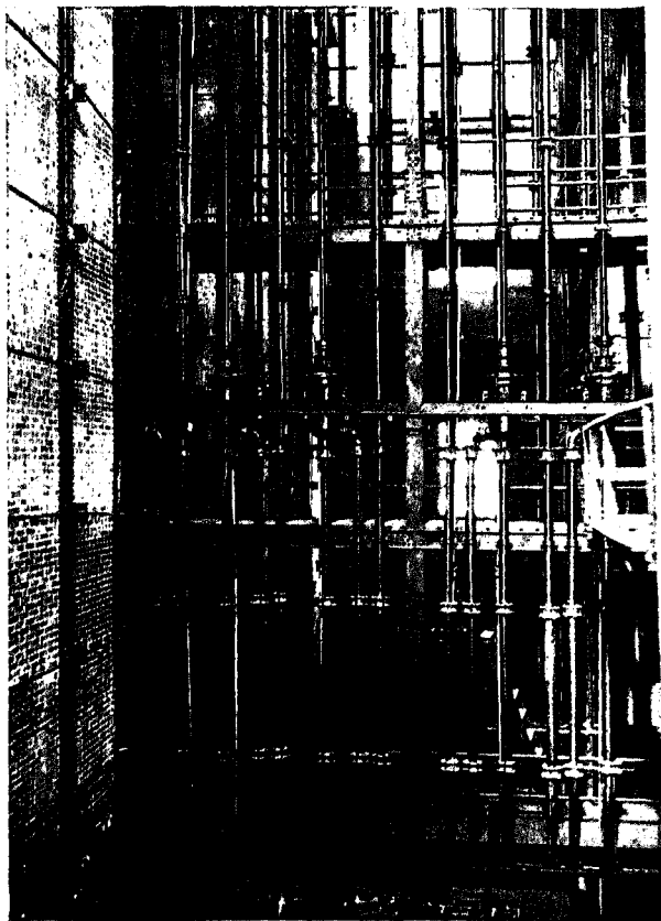
FIG. 121.—Air-lift Installation at Air Nitrates Plant, Muscle Shoals, Alabama, U.S.A. Sullivan Machinery Co.
